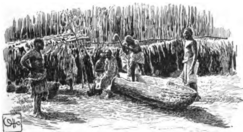
POKOMO BOAT BUILDERS AT WORK
